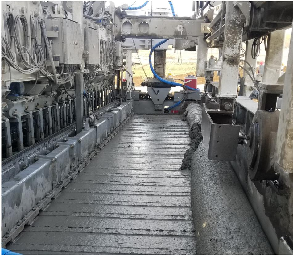
G&Z's DBI accurately inserts dowels in concrete behind the slipform confining pan. The unique combination of the DBI confining pan, trailing sideforms and vibrating forks ensure good consolidation and homogeneous concrete around the inserted dowel bars, even with low airport slump concrete. This is accomplished while minimizing the disturbance to the surrounding concrete surface during insertion.
