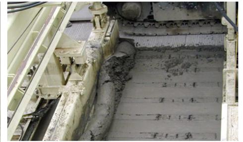
An Oscillating Correcting Beam, which is a part of the DBI System, ensures accurate refining of the concrete surface disturbed by the dowel bar insertion process.
