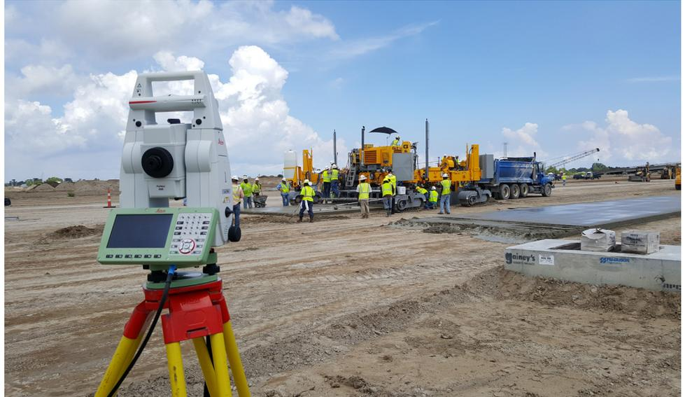
NoLine is comprised of an EGON software upgrade and a hardware mounting kit. EGON NoLine Software Upgrade integrates the use of third-party stringless technology directly into the paver's CAN Bus network.
